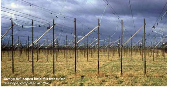
technicians, led by Cambridge University radio astronomer Antony Hewish, had just completed the construction of a sprawling radio telescope near the university: more than 2,000 dipole antennas, lined up like rows of corn and connected by dozens of miles of wire. Jocelyn Bell was one of the laborers: "I like to say that I got my thesis with sledgehammering," she once joked.
