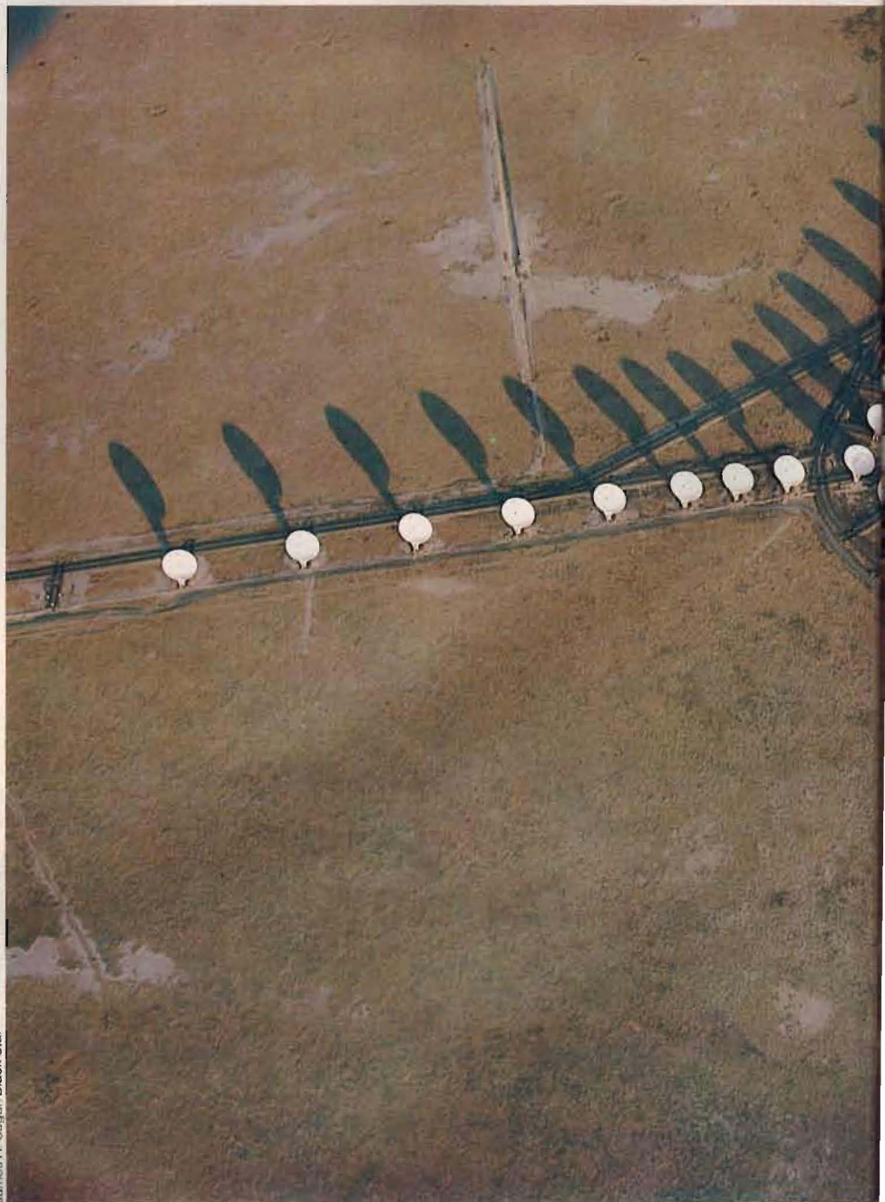
"Mushroom patch": The VLA's 27 antennas can be rolled along tracks to change their configuration. Above, each arm of the "Y" extends about half a mile; this offers a wide-angle view of space. In its most expanded pattern, with each arm reaching 13 miles, the array gives a more closeup view.
